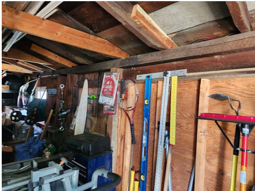
Interior Walls – Replaced Sections and Added Members
