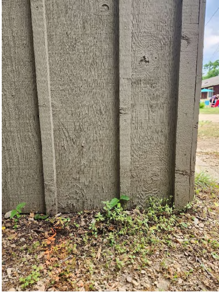
Wood Structure at Grade – Northwest Corner
