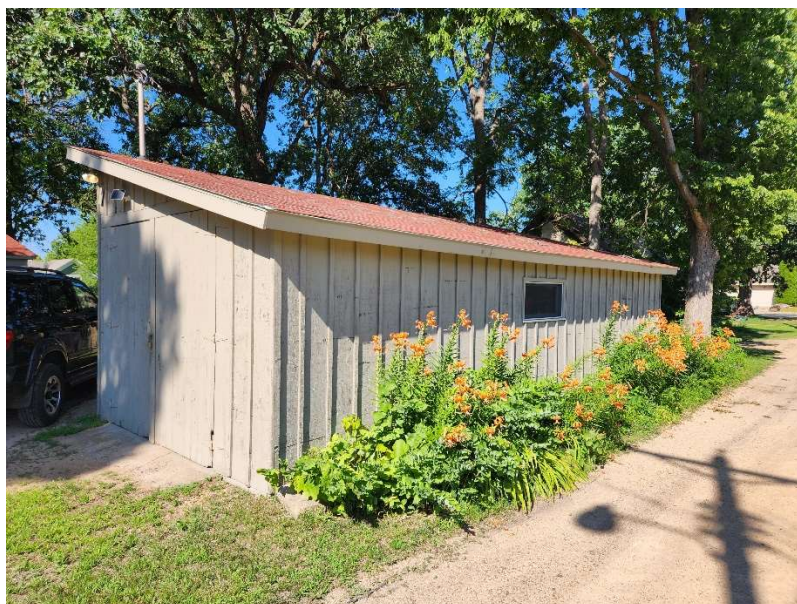
Existing Shed – Viewed From Alley (above)
