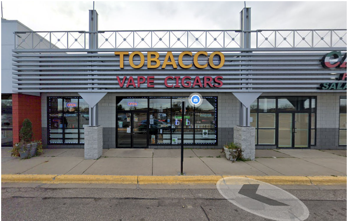
Looking south from front parking lot off 12 th St. W
