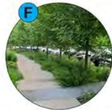
F Parking Lot Runoff Water will sheet flow toward the bioswale / rain gardens and allow for absorption of 13,000 gallons of water during a one inch rain event. Permeable paving will be explored should the capacity of the rain gardens be maximized.
