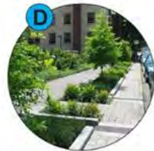
D Road Runoff Approximately 14,000 SF of stormwater runoff from Second Street and Lock and Dam Road can be diverted into tree wells and bioswales. During a one-inch rain event, potential capture could be 7,800 gallons.
