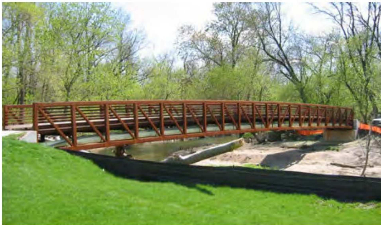
Figure 5: Prefabricated Through Steel Truss
