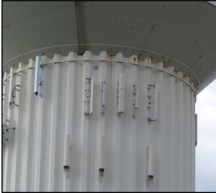
5 'X' SECTOR ANTENNA MOUNT PHOTO SCALE: NONE
