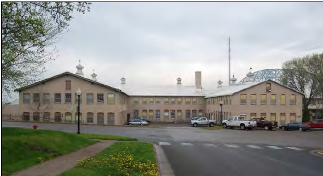
Front of Building of Concern
