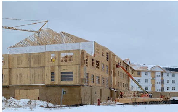
Vermillion Shores Phase II
