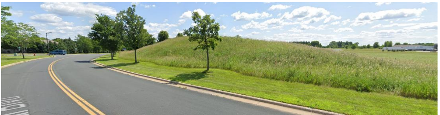
Spiral Blvd. Top soil stockpile recently removed
