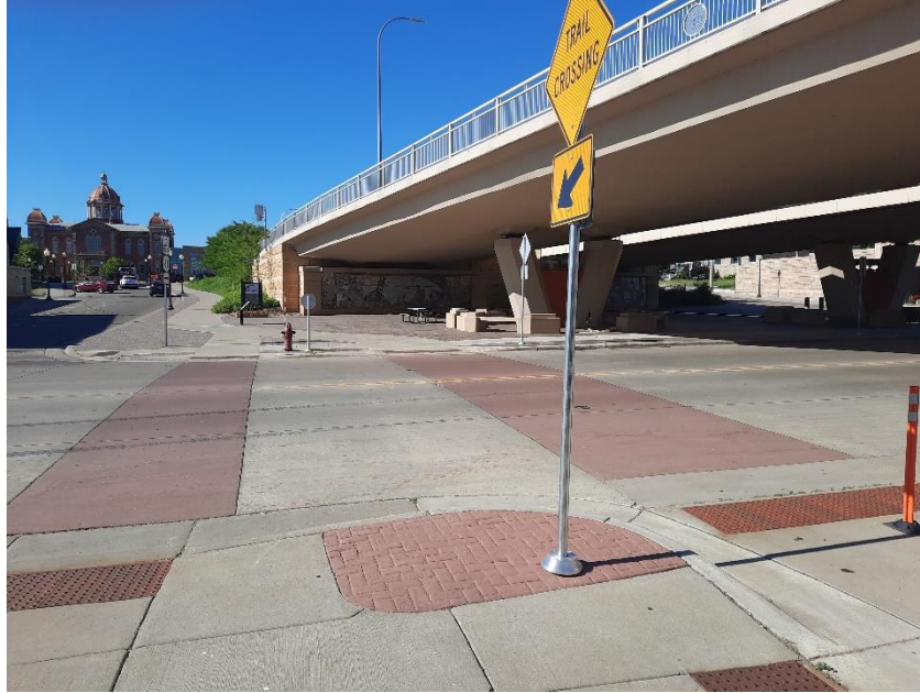
Under the Hastings Bridge – south side
