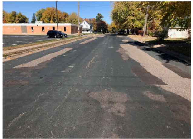
River St – looking north from 4 th St
