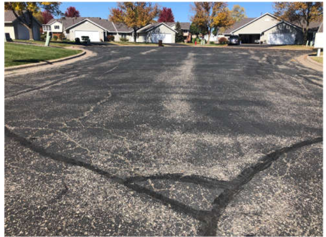
Seton Ct – looking north from 15 th St
