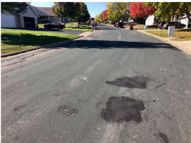
Steeple Ln – looking west from General Sieben Dr
