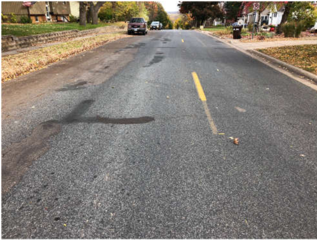
4 th St – looking east from Maple St
