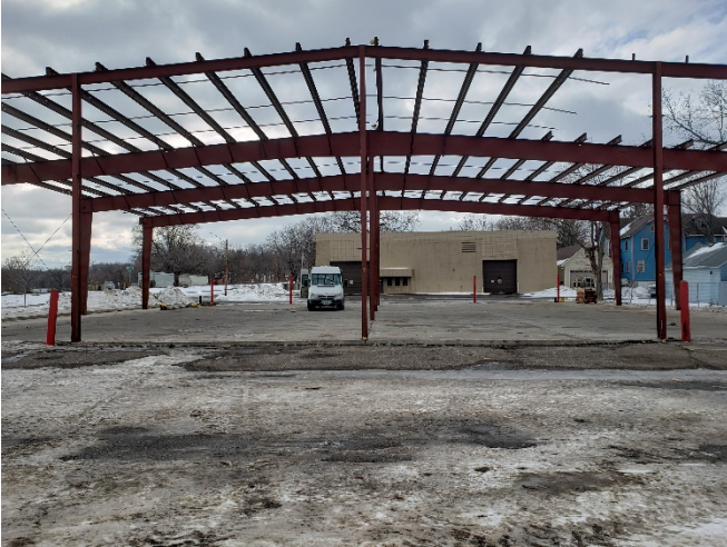
Looking South from 3 rd Street
