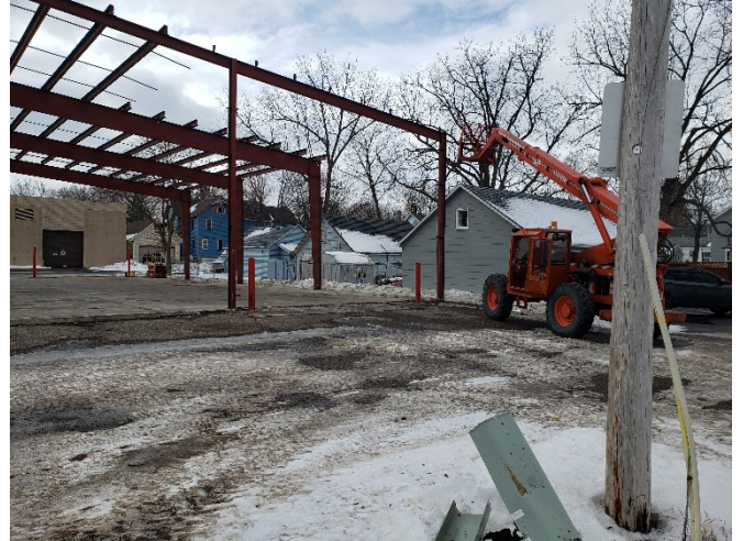
Looking Southwest from 3 rd Street
