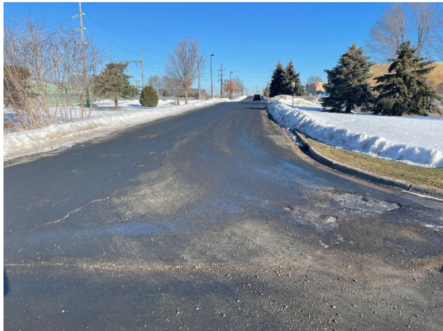
Unnamed Rd – looking north from South Frontage Rd
