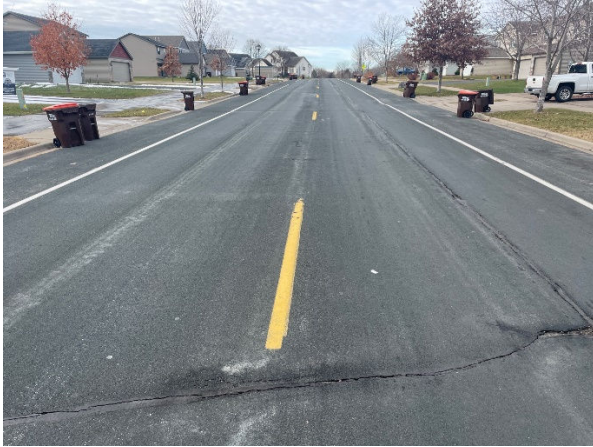
31 st St – looking west from Bohlken Dr
