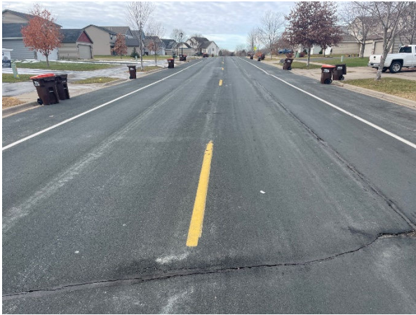
31 st St – looking west from Bohlken Dr
