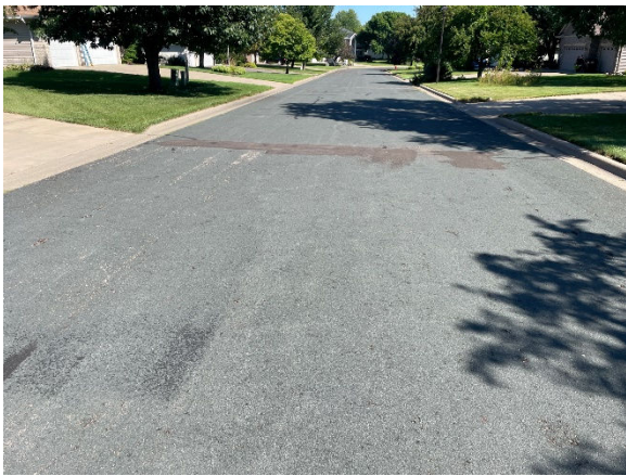
Stonegate Rd – looking north from midblock
