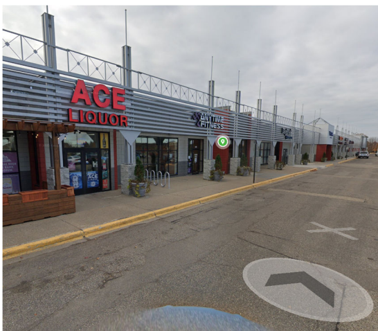
Looking east from the front store parking lot
