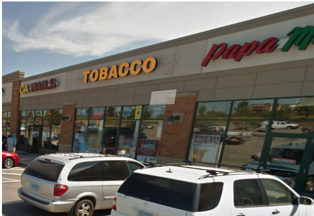
Looking west from front parking lot off South Frontage Rd.
